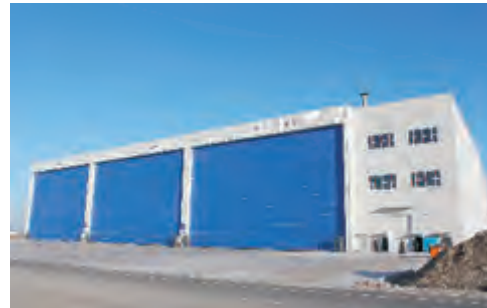
一喷二涂 Painting and Blasting
