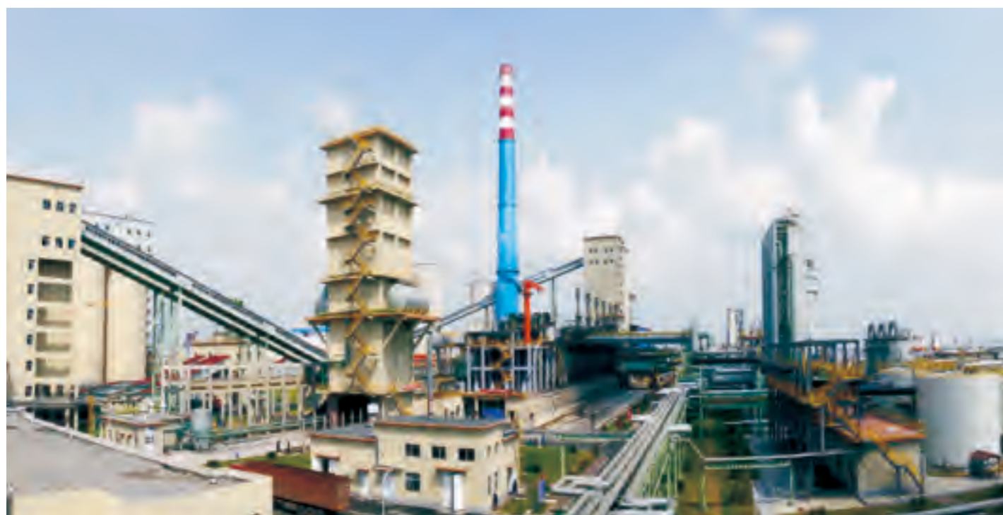
焦化厂全景 Overview of Coking Plant
